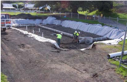
Figures 3 and 4: Sand filter during construction and post-construction showing surcharge above the device
